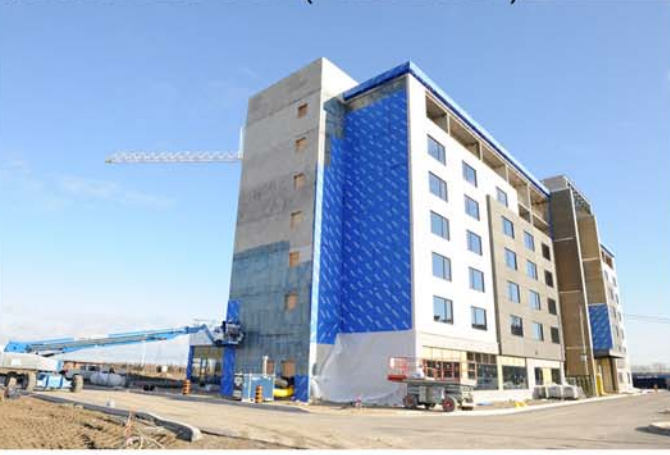
CAMERA VIEW 3 (SOUTH-WEST SIDE)
