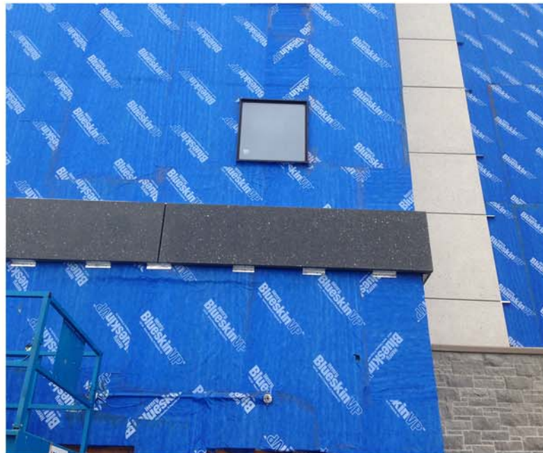
WEST ELEVATION WALL
