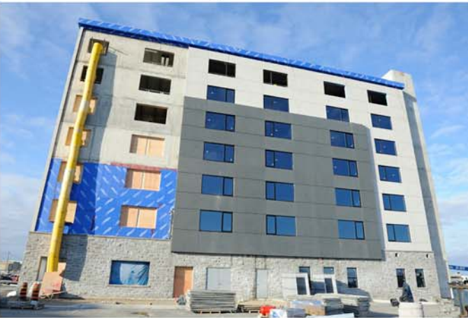
CAMERA VIEW 2 (EAST SIDE)
